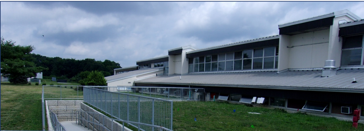
Figure 4 Existing Federal Prison Camp, FCI Danbury
