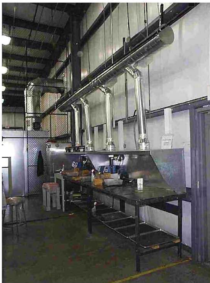
Image 5. LEV hoods and ductwork where chip recovery was performed
