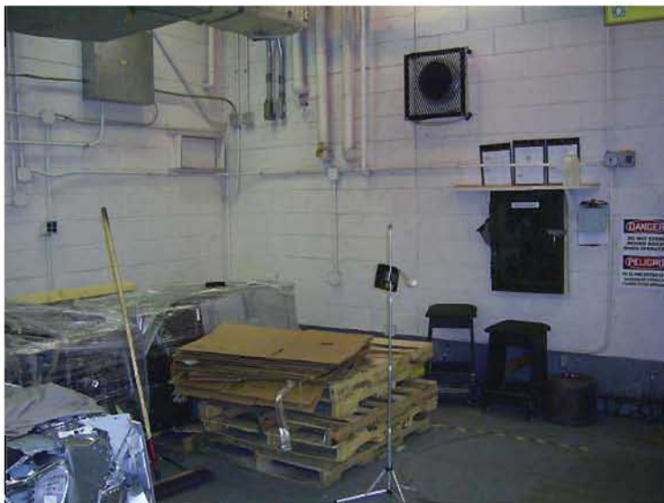
Image 2. Current conditions (January 2008) at the location where CRT glass breaking operations were once performed (glass breaking facilities are no longer there). Note the exhaust air duct in the wall (covered by mesh grille) which leads to the outside bag house as well as the FOH air sampling station in foreground.
